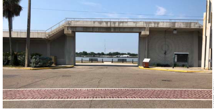
The cobranded seawalls of Morgan City and Berwick provide both necessary resilient infrastructure and a link between the two cities.
